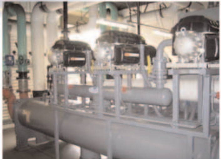
Turbocor compressor installation on existing chiller in Juvenile Hall.
